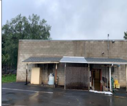
Photo of Fire Station Vehicle Garage
