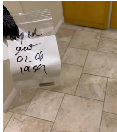
Photo of HA number 19, Sample No. 0206-19-59 | Non-ACM Gray Tile Grout, Within Hallway and Kitchen
