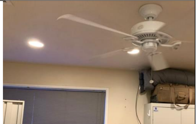
Photo of sample number 28, Non-LBP Drywall Ceiling, Within Bedroom
